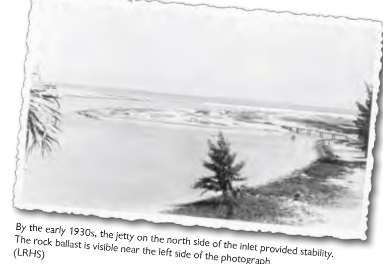
By the early 1930s, the jetty on the north side of the inlet provided stability. The rock ballast is visible near the left side of the photograph. (LRHS)
